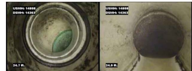
STA 1+26 PIPE BURSTING LIMIT & EXISTING SERVICE LATERAL
